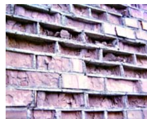
Freeze/Thaw Damage
